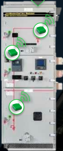
Air Insulated MV Switchgear
