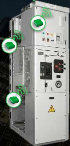
Gas Insulated MV Switchgear
